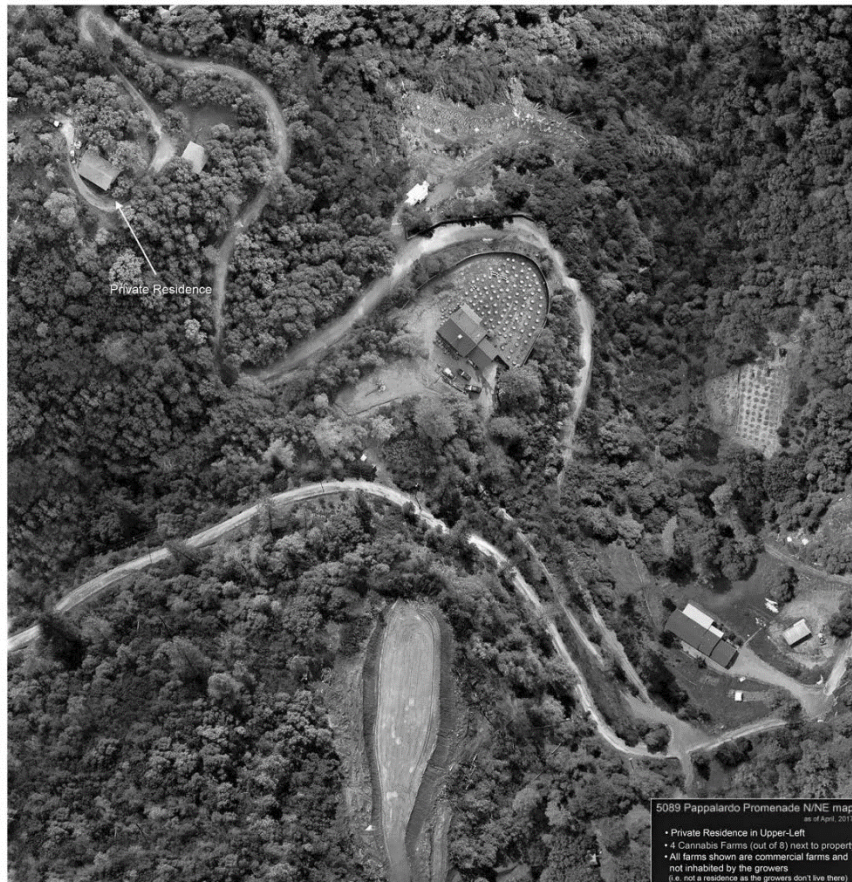
My father's place is in the upper-left. This shows how much excavation has occurred. This picture was taken in May,
